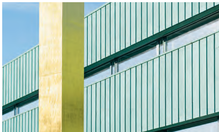
The place with the most accurate measurements in Switzerland: at METAS in Wabern.
